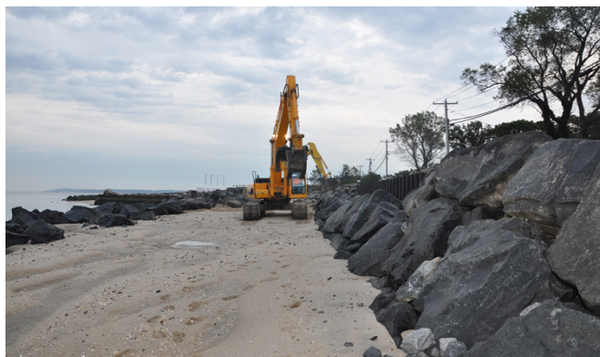
As part of the rehabilitation project a Corps of Engineers contractor places 5 to 7 ton boulders as part of the breakwater. Photo Credit: Dan Desmet, Public Affairs
